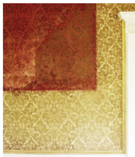
Figure 16 Light damage to the red wallpaper is apparent here in the Red Drawing Room at Uppark House. The red colour has been shielded from the light behind a picture (shown on the right hand side of figure 4). Where the wallpaper has not been covered the red colour has faded to brown. ©NTPL/Andreas von Einsiedel
