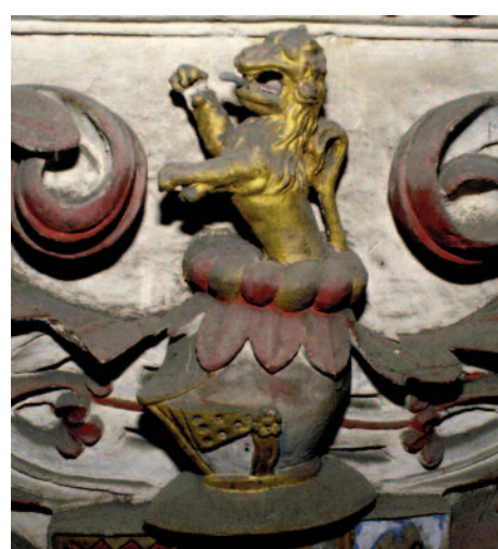
Figure 21 Dust on plasterwork from Chastleton House, Oxfordshire, obscures the original surface finish. Photo: Katy Lithgow
